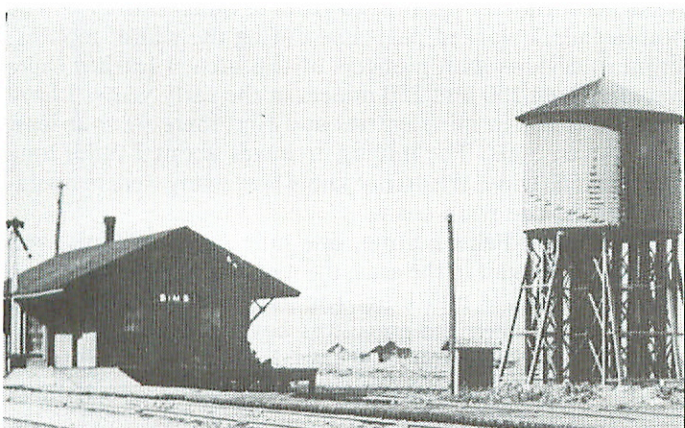
Sims Depot - water tower and water pumping station — about 1915.
